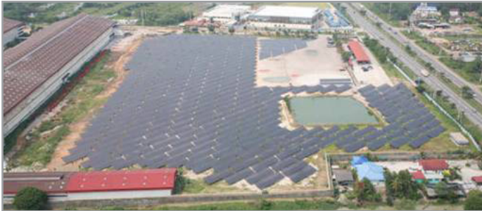
One megawatt solar array in Bangkok, Thailand. An example of the renewable energy development driven by Thailand's VSPP regulations. Photo courtesy of Palang Thai.
