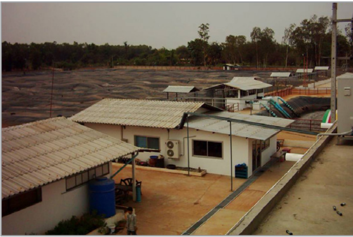
This facility makes methane out of waste water at a tapioca flour plant. Photo courtesy of Palang Thai.
